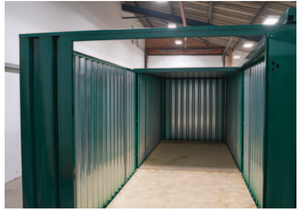
2.21 Slide roof panels up from either end, the ID plates on each roof should be facing outwards.
